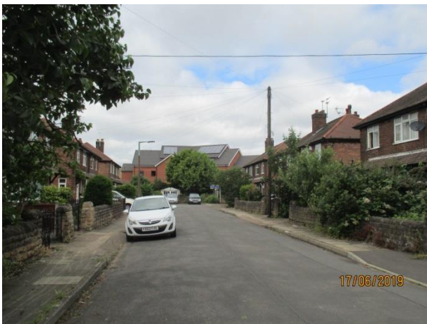
View along Princess Avenue with rear elevation of Flewitt House at the end
