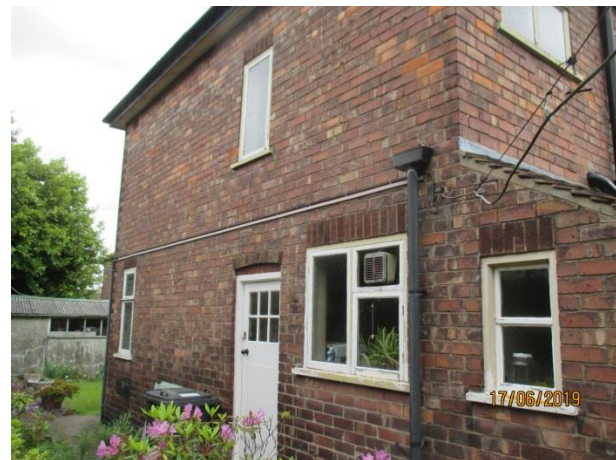
Side elevation of 23 Princess Avenue
